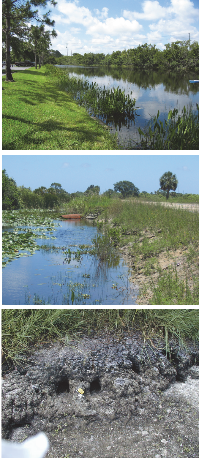
Figure 2. Representative localities: Imperial Hotel retention pond (top); Eau Gallie Ditch (middle); Sotille Canal showing burrow-ridden bank (bottom).
